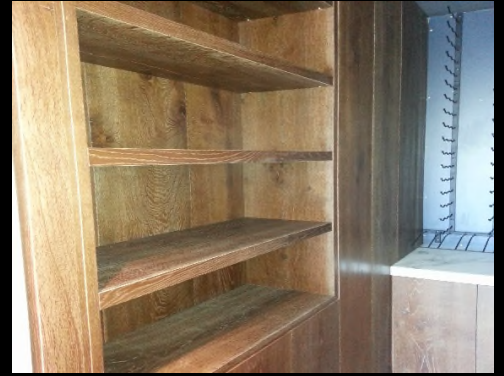
Bookcase constructed with Engineered floor
