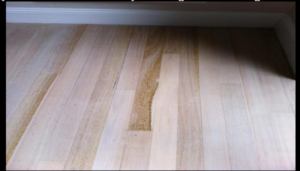
BLACKBUTT TANNIN SHOWING AFTER CLEAR COAT
