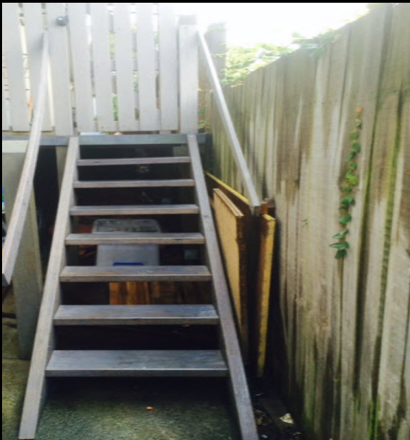
F17 Hardwood External open staircase
