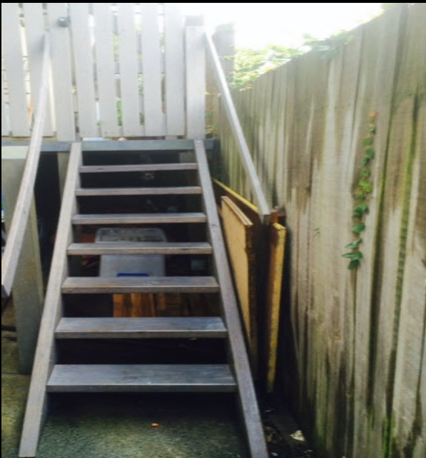
F17 Hardwood External open staircase
