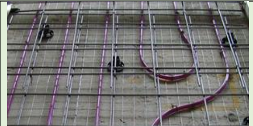
Pipes in concrete
