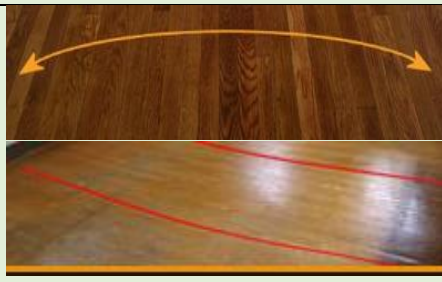
Sand level old floor
