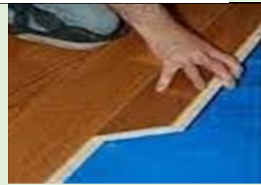
Concrete → Underlay → Floor
