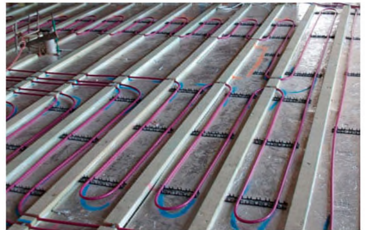
^^ Between Batten Installation ^^
