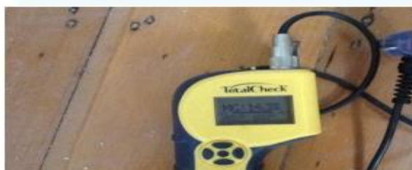
Moisture meter- Sub Floor testing at 14.3% (unable to install as MC variation is 3.2%)
