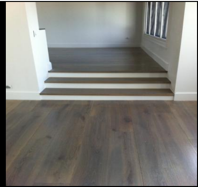
Stained staircase to match floor
