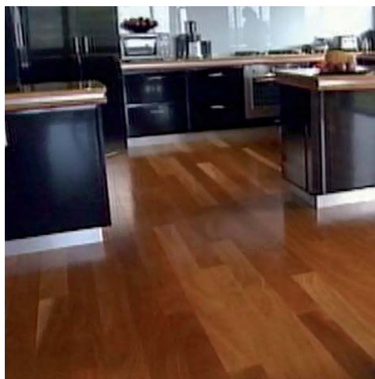
A completed site sanded and coated floor
