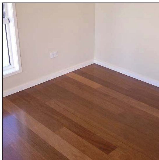
Site sanded and coated engineered floor
