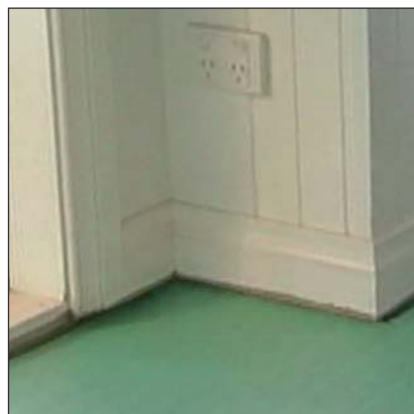
Underlay is cut neatly around corners
