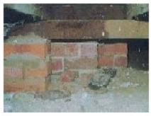
Moisture may be trapped at various points in the sub-floor. Earth may build up arround the perimeter of the house (particularly in old houses) so the sub-floor is effectively dammed.
