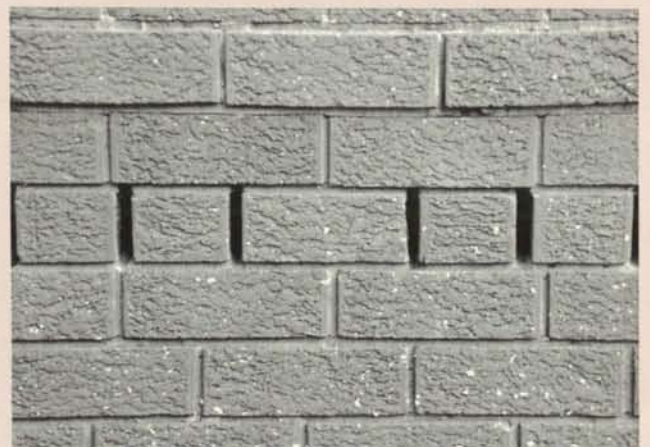
Figure 5. Spaced brick ventilation.
